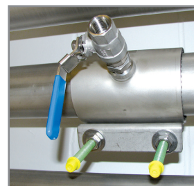
B Spot drilling collars
